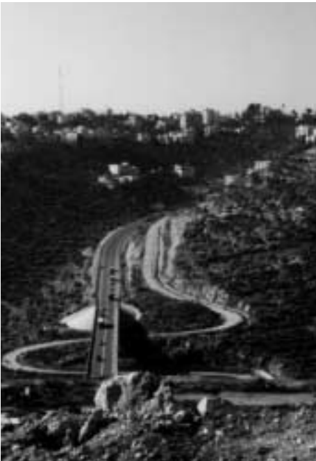
Bypass road bridging over dilapidated Palestinian road between Gilo and Beit Jala
